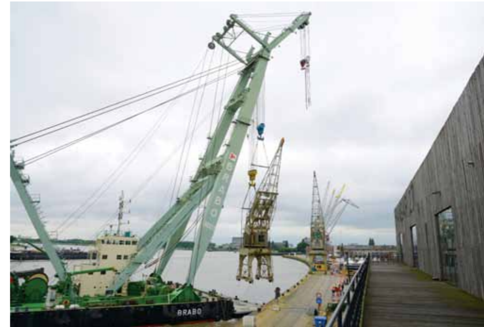
On the move: the 800-tonne floating crane Brabo gives one of the old cranes a new place on the banks of the Scheldt.
